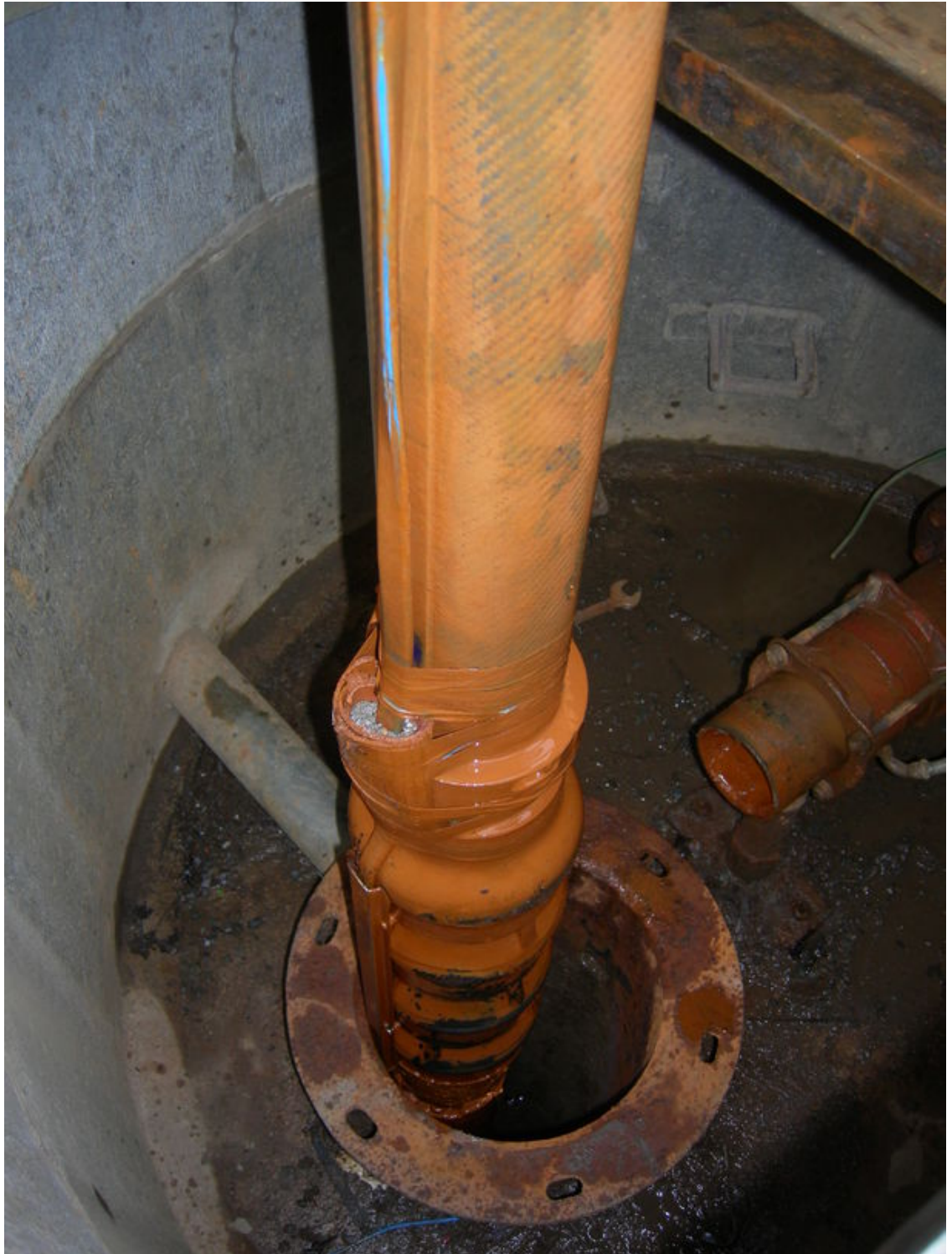
If left unchecked iron bacteria can build up on water pumping equipment
